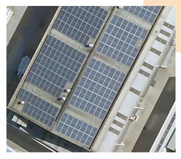
System Size: 70.56kW Location: Lansvale, NSW Panels: 196 X Trina 360W Inverter: 2 x Solaredge 27.6kW
